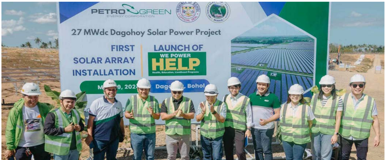
PGEC and Dagohoy Green Energy Corporation (DGEC) held the first solar array installation for its 27MWdc Dagohoy Solar Power Project (DSPP) last May 9, 2024. The event was attended by Bohol Gov. Aris Aumentado (5th from left) and key leaders of the province of Bohol and municipality of Dagohoy, officials from the National Grid Corporation of the Philippines (NGCP), and various stakeholders.
